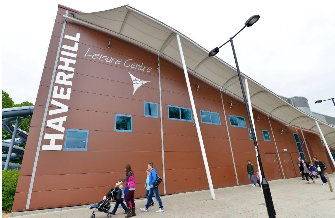
Haverhill Leisure Centre
